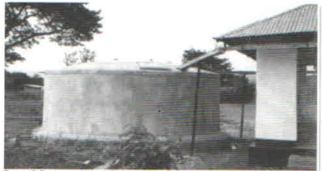
Figure 12. Ferrocement tank in Ruganzu Village ©OTU
